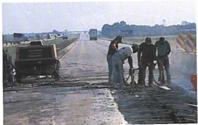
Figure 10-23. Door closers and air tools are examples of open pneumatic systems, since they use atmospheric air in their systems.
