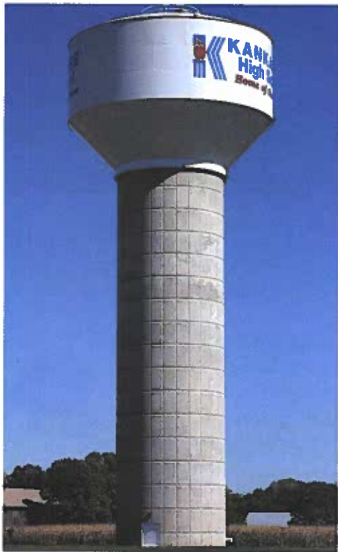
Figure 10-4. The type of water tanks used by communities to store water and provide good flow into water taps must be built to withstand tremendous pressure due to the weight of the water stored in them.
