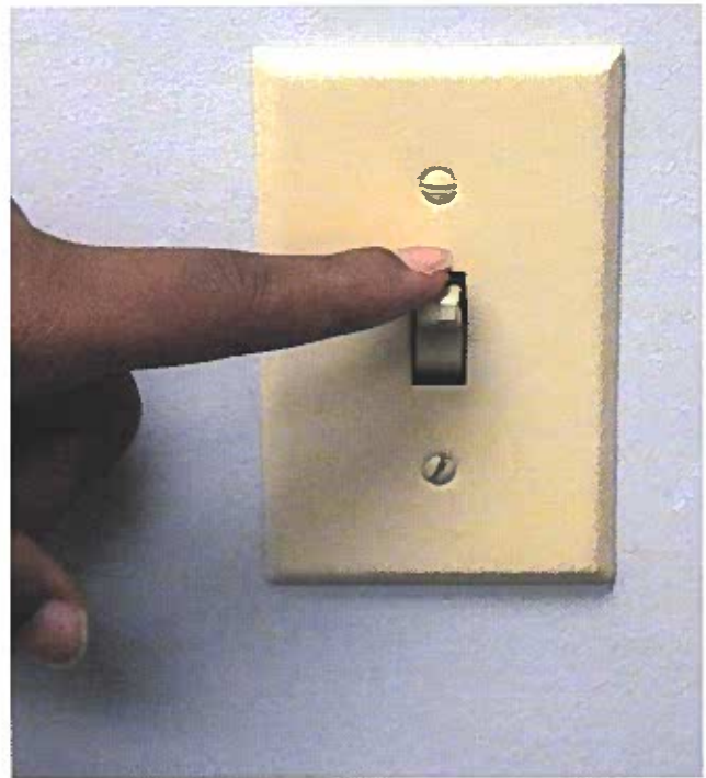
Figure 11-5. A light switch is an example of an open loop control system. There is no feedback to indicate whether the lamp did or did not turn on.
