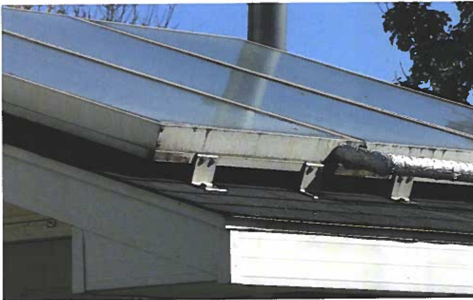
Figure 13-20. An active solar energy collector system performs a frequency conversion, changing visible light into infrared energy.
