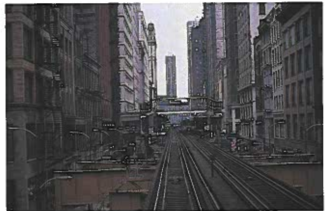
Figure 17-26. The "El" is Chicago's elevated railway system, which encircles the downtown area one story above the street. Although these systems can be used with light-rail vehicles, it is more common to use heavy-rail trains. Note the massive beams supporting the rail structure.
