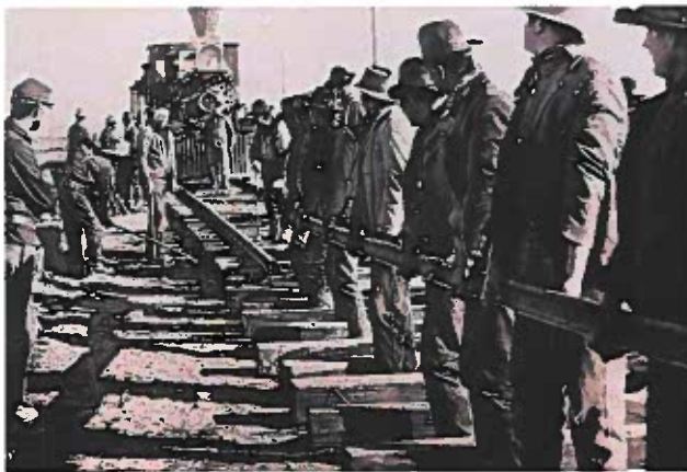
Figure 17-5. This photograph commemorates the laying of the last section of track that linked the East and the West. (Burlington Northern Santa Fe)
