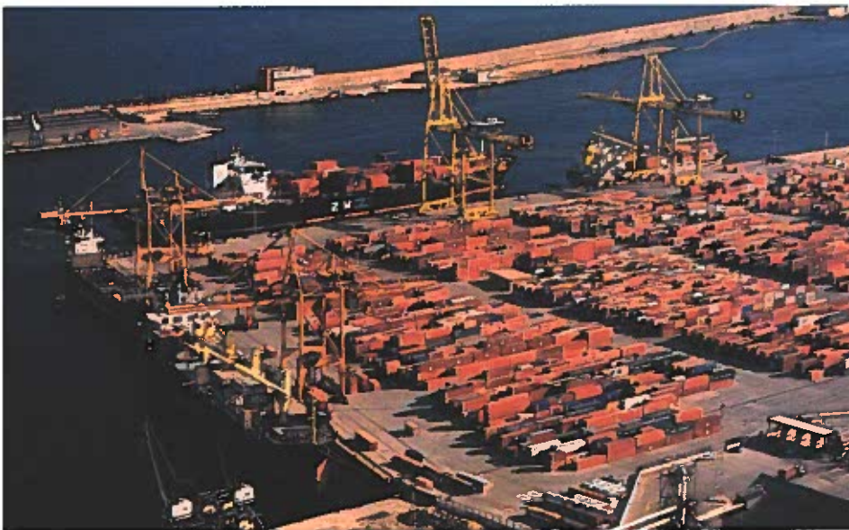
Figure 25-3. This port facility is an example of intermodal transportation. Shipping containers arriving onboard the ships are unloaded and stored before being transferred to railcars or truck chassis to continue their journey. Movement in the opposite direction also takes place. Containers arriving by rail or highway are stored and then loaded onto ships.
