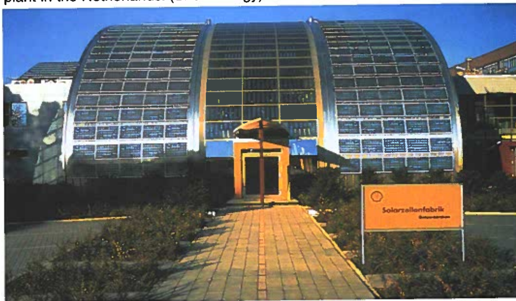
Figure 27-3. Photovoltaic cells are seeing increasing use as an alternative energy source. This large array covers the roof of a solar cell manufacturing plant in the Netherlands. (Shell Energy)
