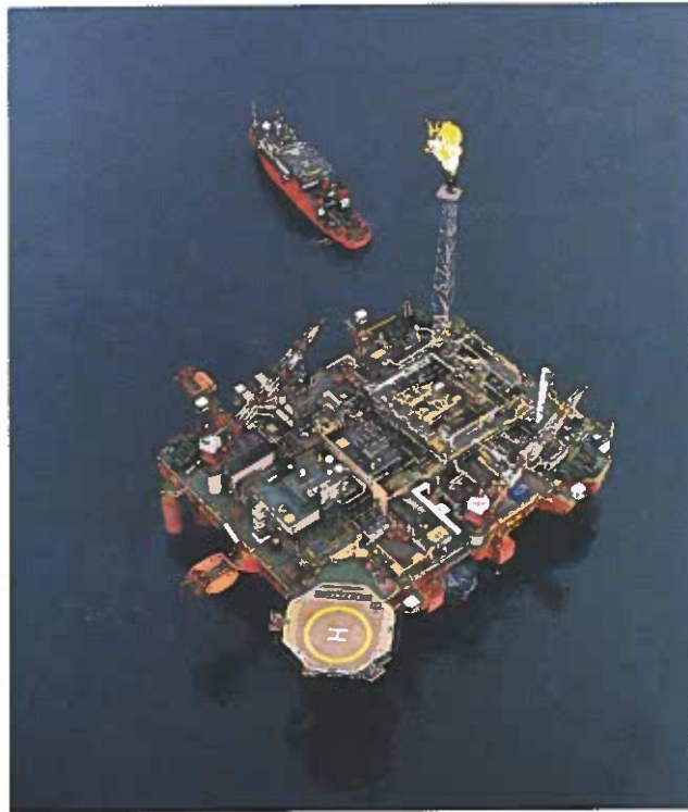
Figure 3-9. Oil is extracted from formations beneath the land and oceans by drilling into the formations and pumping the oil to the surface for transport by ship or pipeline. This is a large floating platform anchored over a well in England’s North Sea oil field. (Kerr-McGee Corporation)
