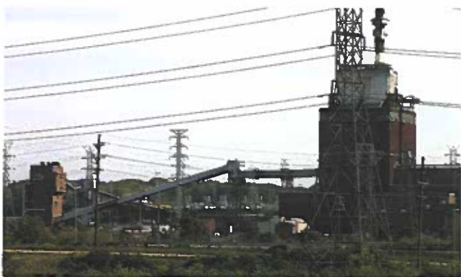
Figure 3-2. A large number of electrical generating plants burn coal to generate steam that drives the turbines.
