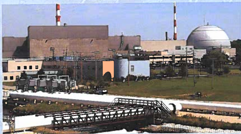
Figure 4-A. Dresden I, a commercial nuclear reactor, opened in 1959 in Morris, Illinois, west of Chicago. The unit was retired from active service in 1978, although two later units remain in operation at the same site. The spherical object is the containment structure of the Dresden I reactor. (Exelon Energy)
