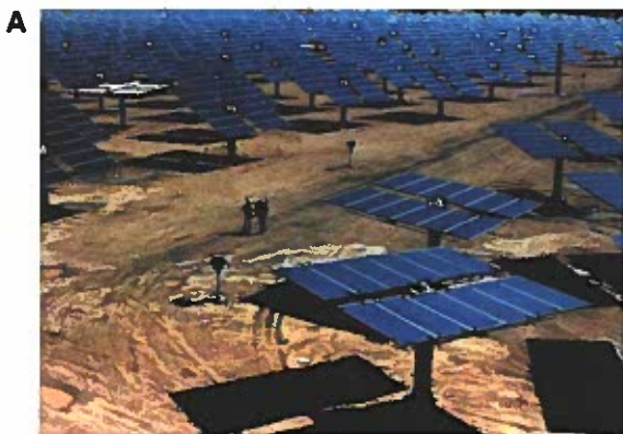
Figure 6-18. Solar Thermal Energy Conversion (STEC) is an experimental program being evaluated at the Sandia National Laboratory of the Department of Energy (DOE) in New Mexico. A—Nearly 2000 large mirrors are arranged in an arc across 72 acres and are kept oriented to the sun. B—Sunlight reflected from the mirrors is focused on a receiver near the top of a tall tower. The resulting heat energy is used to generate steam and drive a turbine. Electrical energy to power 10,000 homes is generated by this system. (U.S. DOE)
