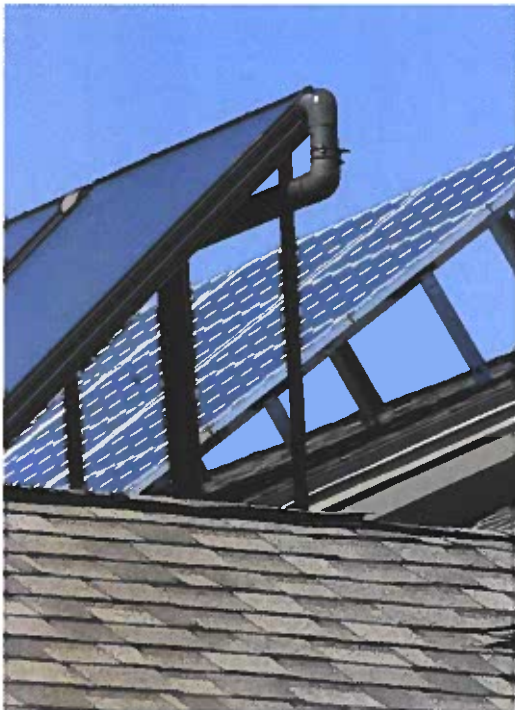
Figure 6-1. Solar energy can be captured to provide heating or electrical power for a structure. Two different capture methods are being used in this home, which was designed to make extensive use of solar energy. The flat-plate collector on the left captures solar energy and uses it to heat water for household uses. The photovoltaic panels on the right convert the sun's energy to electricity, which is then stored in batteries for later use.
