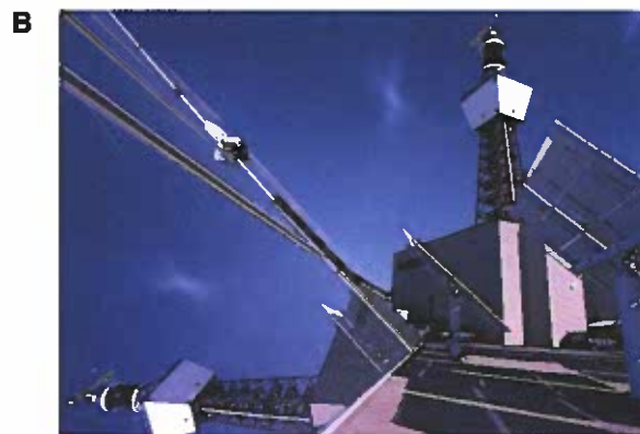
Figure 6-18. Solar Thermal Energy Conversion (STEC) is an experimental program being evaluated at the Sandia National Laboratory of the Department of Energy (DOE) in New Mexico. A—Nearly 2000 large mirrors are arranged in an arc across 72 acres and are kept oriented to the sun. B—Sunlight reflected from the mirrors is focused on a receiver near the top of a tall tower. The resulting heat energy is used to generate steam and drive a turbine. Electrical energy to power 10,000 homes is generated by this system. (U.S. DOE)
