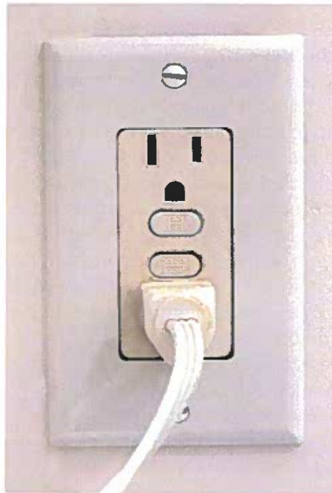
Figure 8-42. Ground Fault Circuit Interrupters (GFCI) are designed to protect people from electrical shock. A—A typical GFCI used in a bathroom or other location within 6' of a sink or other water source. B—The GFCI uses a sensing circuit to detect an imbalance between current flowing in the hot and neutral sides of the circuit.
