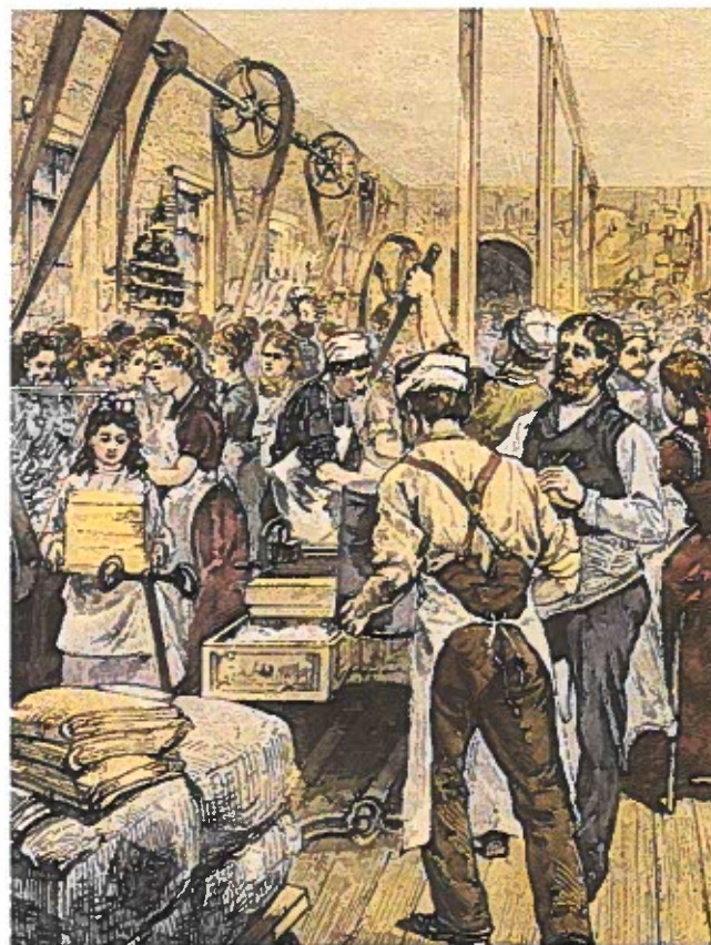
Fig. 2-5. By the late 1800s, entire factories were powered by steam. In this textile factory, an overhead shaft and belt system allowed a single steam engine to run every machine in the factory.
