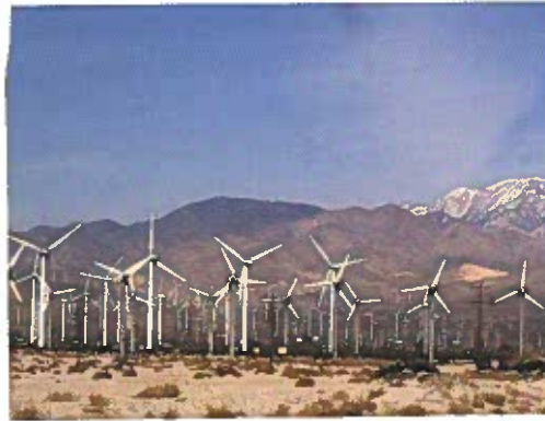
Figure 10-25. Wind turbines on a wind farm capture the kinetic energy in surface winds and convert it into electrical energy in the form of electricity.
