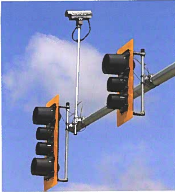
Figure 12-45. In many cities, traffic signals are enforced by security cameras. The cameras are programmed to take pictures of vehicles that fail to obey stoplights.
