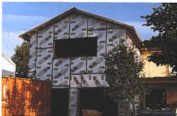
Figure 4-4. Insulating materials help slow the passage of heat or cold through walls of homes.
