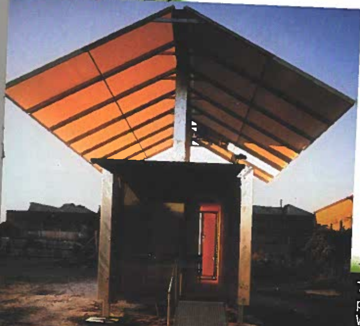
A shipping container provides the basis for a self-contained refugee housing unit.
