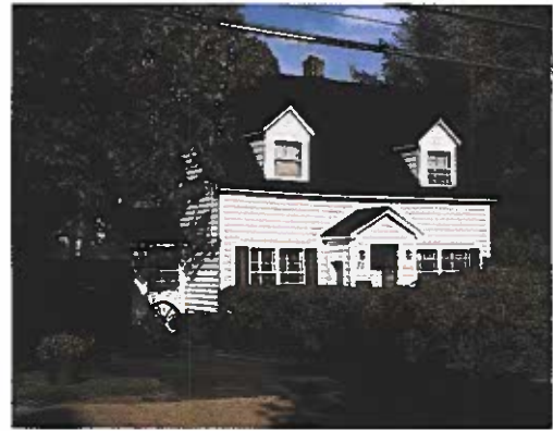
Figure 7-7. In a one-and-a-half story home, the rooms on the second level extend into the roof.
