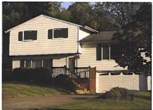
Figure 7-9. A split-level home is divided vertically. The floors of one part of the house are located midway between the floors of the other part.
