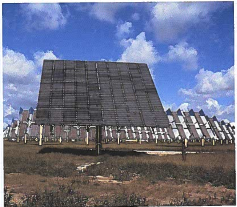
Fig. A. Here, large groups of photovoltaic cells convert solar energy into electrical energy. "Solar farms" like this may become major sources of electricity in the future.
