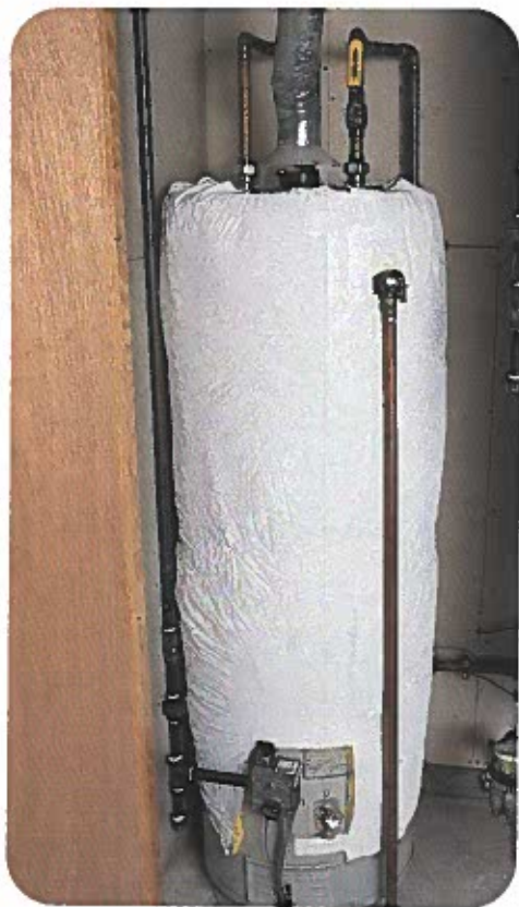
Fig. 13-6. Wrapping a water heater with insulation saves energy. Stop at an appliance store and look at the EnergyGuide stickers that show how much energy a large appliance saves. Describe the stickers to the class.
