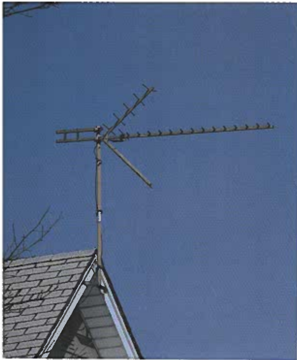
Fig. 16-2. An antenna receives a TV signal and transmits it through wires to the receiver inside the house.
