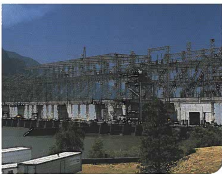
Fig. 7-2. Electricity produced by this hydroelectric plant on the Columbia River in the Pacific Northwest is renewable. As long as the river flows, its energy can be gathered and used. Many people are concerned about the effects of dams on the environment. Research the pros and cons of dams and hold a class debate on the issue.
